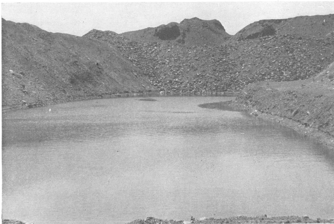
FIGURE 49.—Orchard No. 2-bed stripping, near Mary D Village, Southern field (carbonaceous slate and coal in spoil bank).
